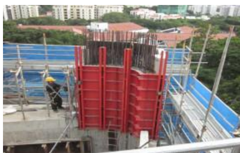
Ván khuôn thép cột dạng cong/ Curved Shaped Column Steel Form
